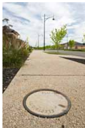
Left, the pit lid rings are made of the same material that the pits are made of and are attached with glue and/or screws
